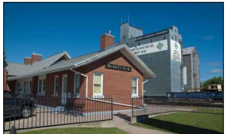
Grain elevators dominate the Sleepy Eye skyline. This one is located near the utility, north of and across the tracks from the museum.
