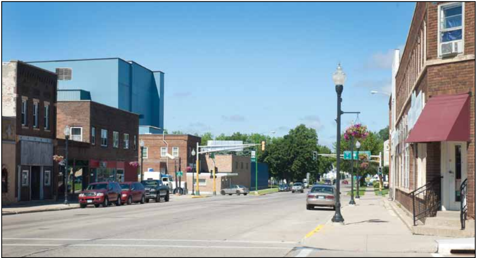
The Sleepy Eye 'main drag' boasts a number of classic two-story brick buildings, although businesses to fill them are hard to come by.
